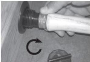
7. Thread hose onto the spa drain.
